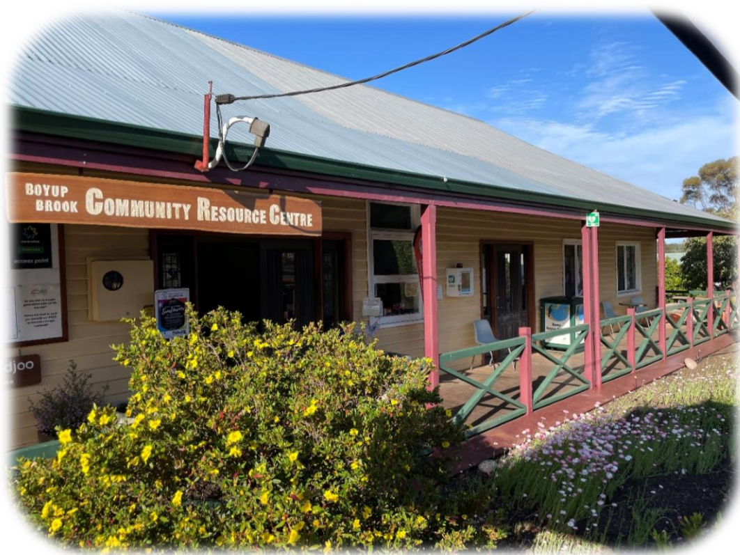
Boyup Brook Community Resource Centre frontage
